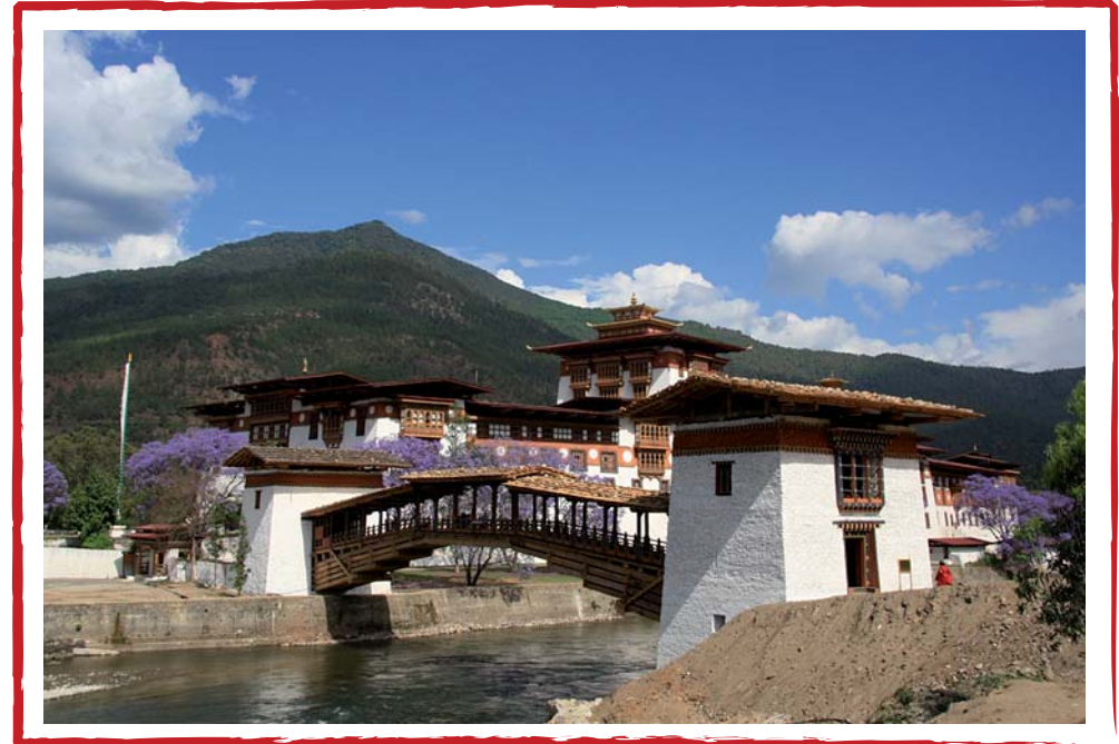
New bridge seen from Punakha village, 10. May 2008
